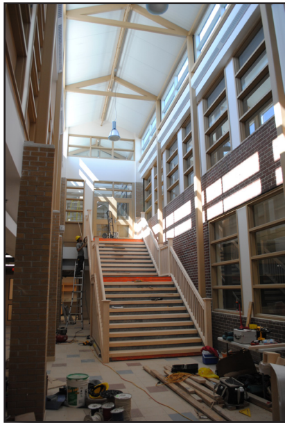
Renovation construction at Hillcrest Public School
